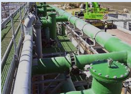
Oil/Gas Leak Detection
